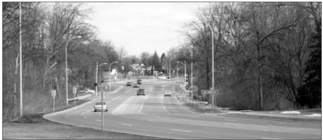
Whitetopping, a concrete overlay containing Blast Furnace Slag, tops Outer Drive in Dearborn, Wayne County, Michigan.
